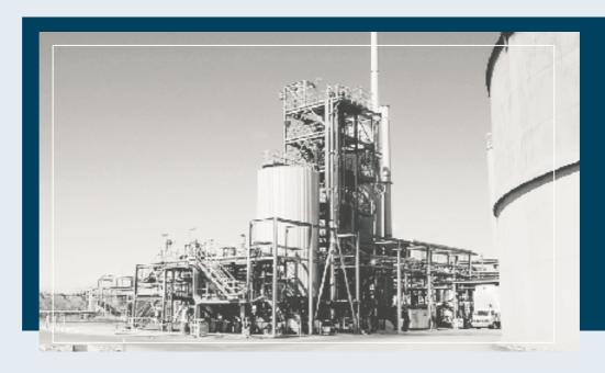
Tiwest's Synthetic Rutile Plant in Kwinana has made significant eco-efficiency gains since it began in 1991. In an example of industrial ecology, waste hydrocholoric acid is converted by a neighbouring company into ammonium chloride for use at another Tiwest operation which supplies the pigment plant.
